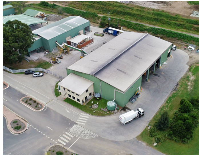
Above: The Materials Recovery Facility at the Tuncurry Waste Management Centre.
