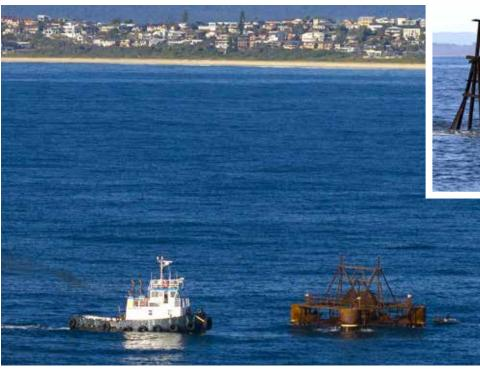
Above: The artificial reef module was pulled into place 4km from the Forster Tuncurry channel entrance before being sunk (photo at top right) to create a reef on the sandy ocean floor 30-35 metres below. One Mile Beach in Forster is in the background.
