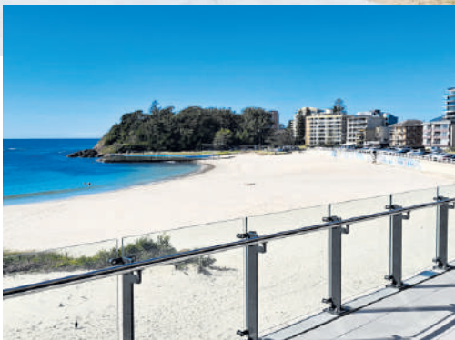
Above: The new Forster Surf Club house and grand view from the upper deck.
