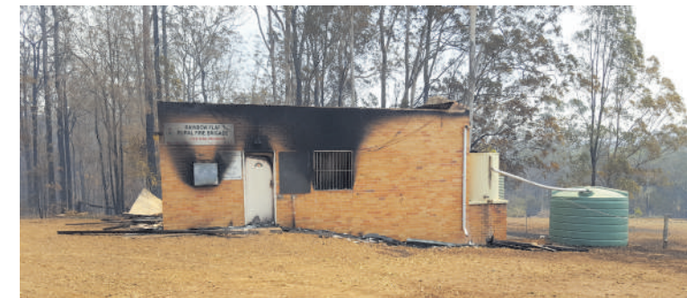
Left: Rainbow Flat RFS Station destroyed by fire.
