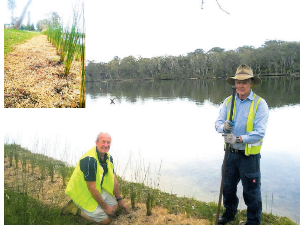
Above: John Marshall from Dads Army/Navy and Steve Howard from Mid Coast Council planting rushes along the banks at Elizabeth Reserve to help prevent erosion. Photos supplied.
