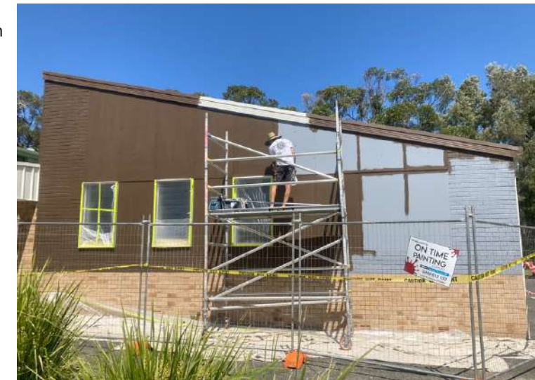
Above: Painting the new Forster Gallery facade.
