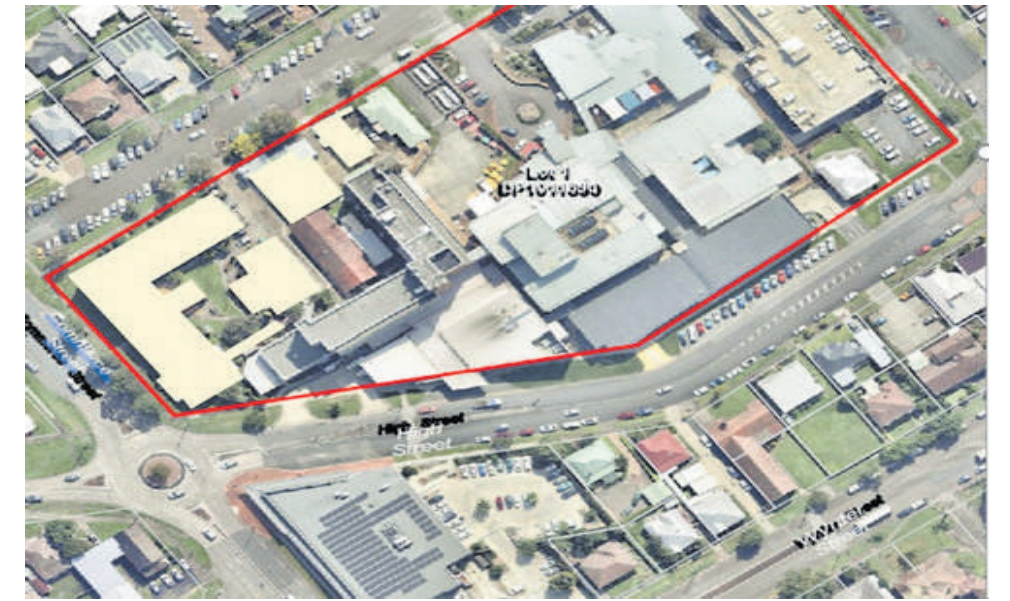
Above: Aerial photo showing the buildings within the Manning Base Hospital boundaries in red. The four buildings highlighted in beige are proposed to be demolished in the early works for Stage 2 Redevelopment.
