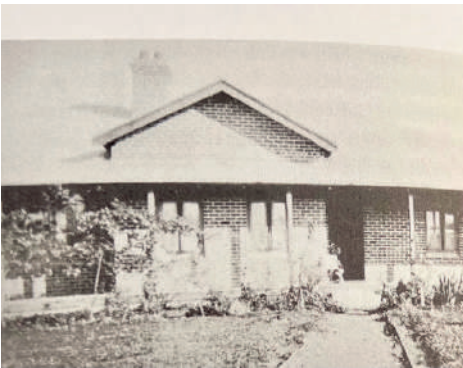
Above: John Milliken’s homestead that still stands at 912 The Lakes Way.
