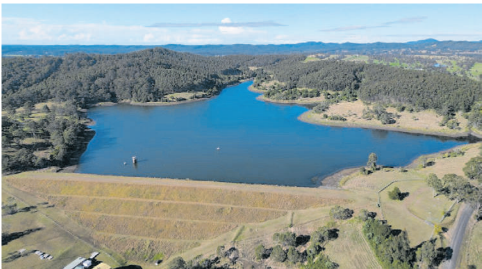
Above: Urgent work will take place to restore the damaged section of the water pipeline that crosses the Manning River between Bootawa Dam and Wingham reservoirs.
