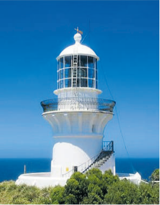
Above: Sugar Loaf Lighthouse at Seals Rock.
