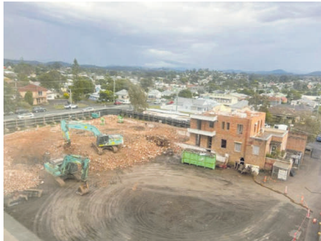
Above: This third photo shows the last part to be demolished once the gas tanks are moved. The angle of this photo is slightly different but the remaining building on the far right (with white balconies) can be seen in each photo.
