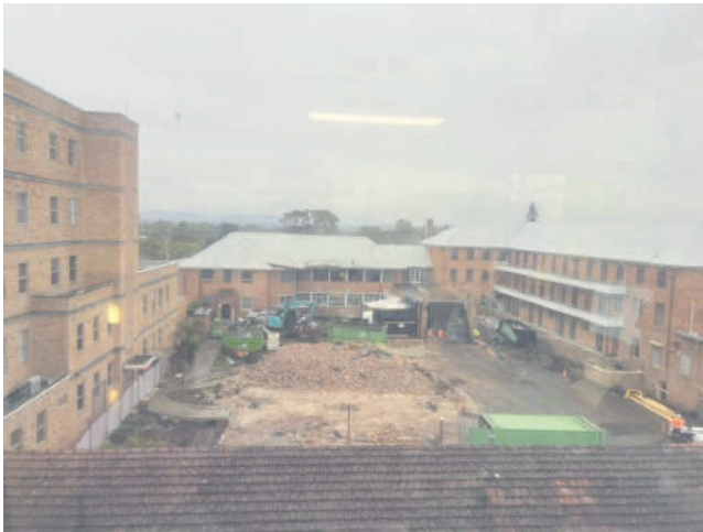
Above: This photo is of much the same angle. It shows that the old fever ward has been demolished. Photos supplied.
