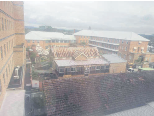
Above: These three photos show the progress of demolition work ready for more Stage 2 Redevelopment. The rusty old building in this photo was the old fever ward.
