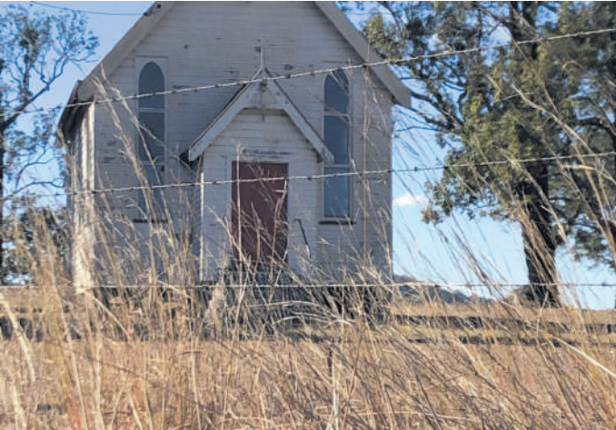
Left: Krambach Presbyterian Church. Image credit MidCoast Council
