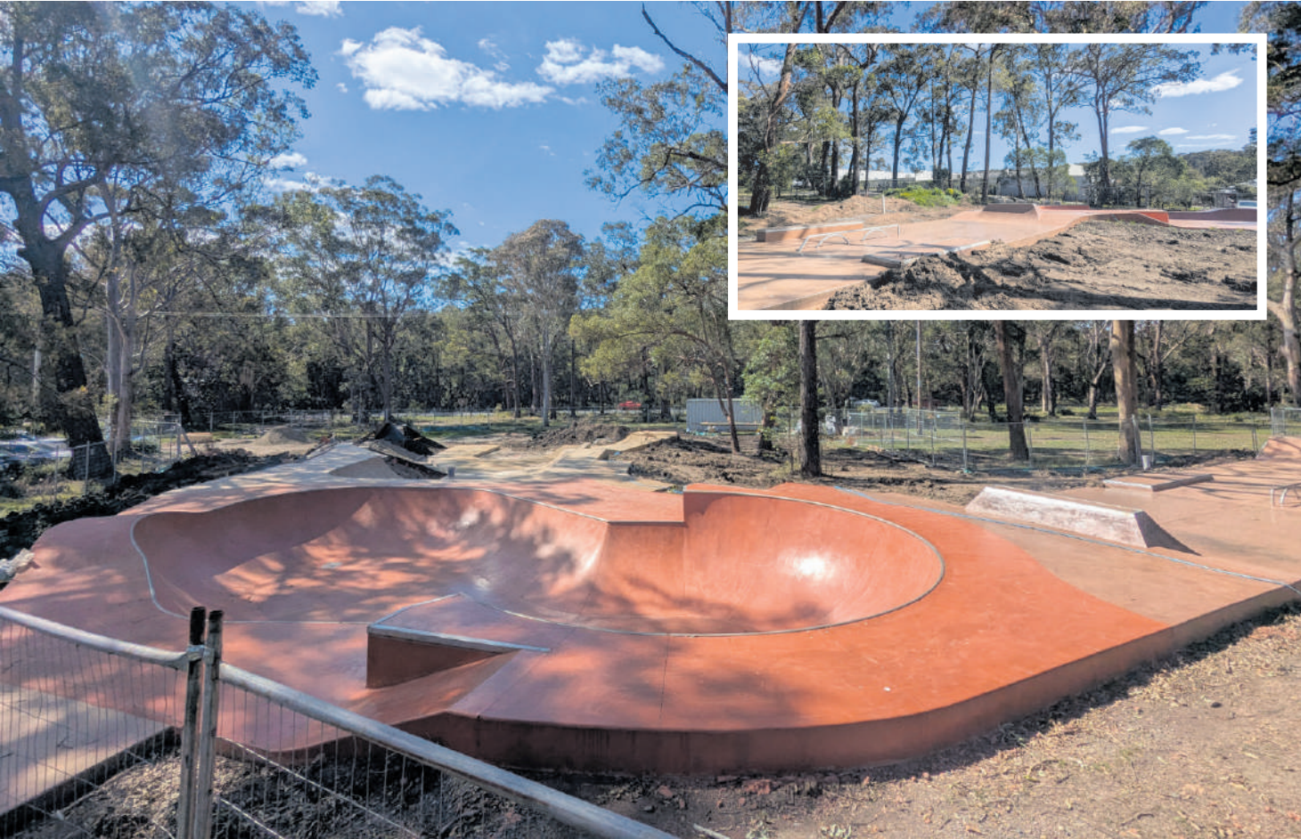
Above: Photos from Sunday 30 August showing great progress of the new Hallidays Point Skatepark, by Matilda Yule.
