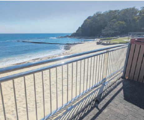
Above: Section of new fencing at Main Beach. Photo by Mary Yule.
