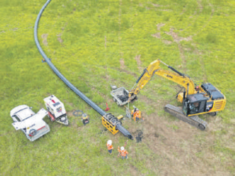
Above: Manning River Underbore.
