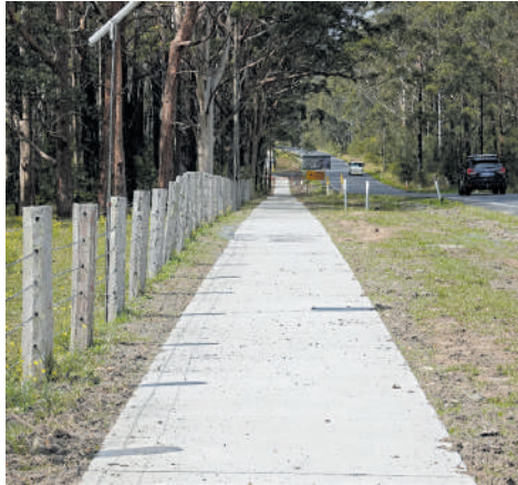
Above: The Black Head Road Pathway is expected to be completed in June.
